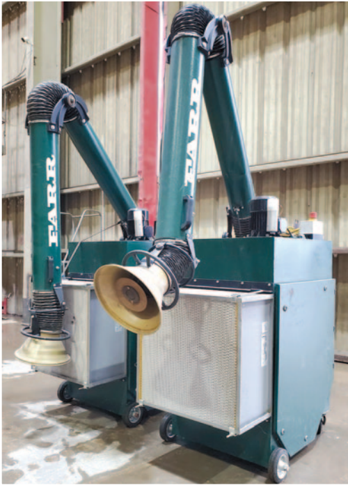
• View of Farr Welding Dust Collectors
