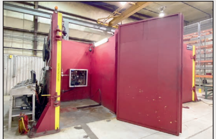
INSIDE VIEW OF BUNKER
