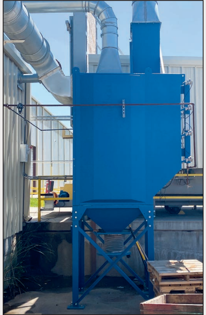
TORIT DONALDSON DUST COLLECTOR
