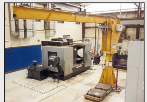
(2) FLOOR MOUNTED AND (20) COLUMN MOUNTED JIB CRANES
