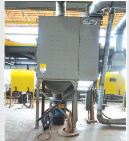
UAS Dust Collector for Pedinghaus Plate Processor
