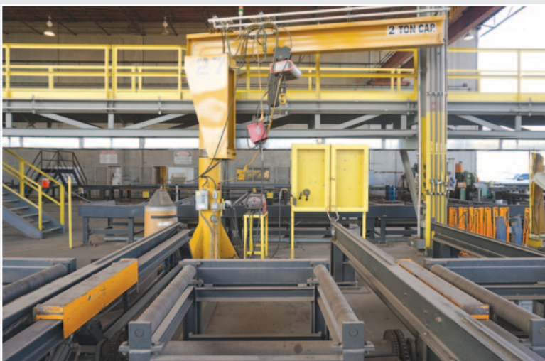
View of Welding Stations To be Sold: Jib Crane, Welding Power Source, Feeder & Tool Box All Together
