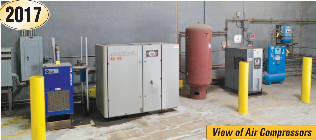
Mattei AC45 HHX 60 HP Compressor with Beko Mdl. RAX300 Air Dryer
